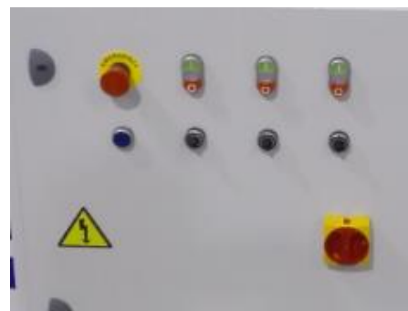
PANEL DE CONTROL/ CONTROL MACHINE
