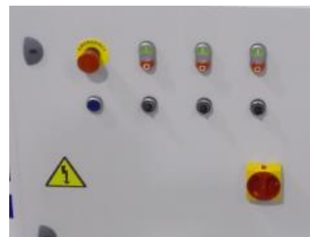
PANEL DE CONTROL/ CONTROL MACHINE
